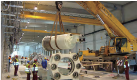
Transfer and installation of extrusion presses
