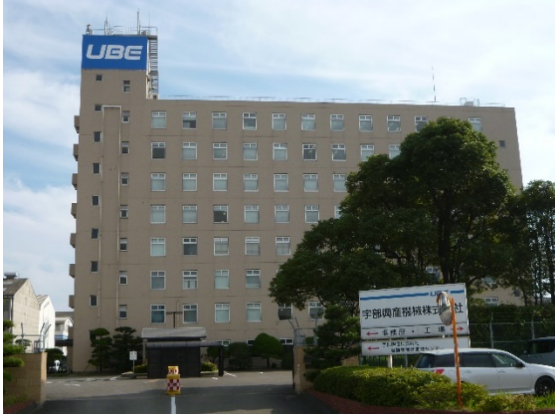
Ube Head Office of Ube Machinery Corporation, Ltd.
