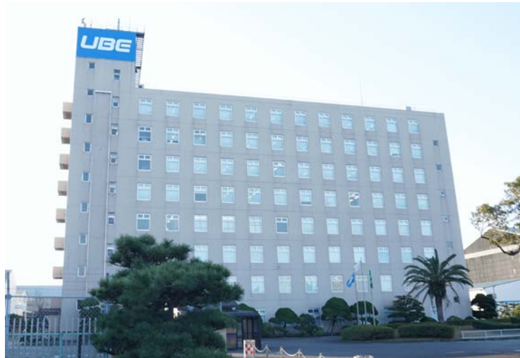
Head Office of UBE MACHINERY
