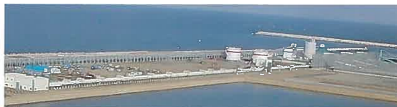
1,100t/h エア浮上コンベヤ (縦二重管式) 1,100t/h Air Floating Conveyor (vertical twin-pipe type)
